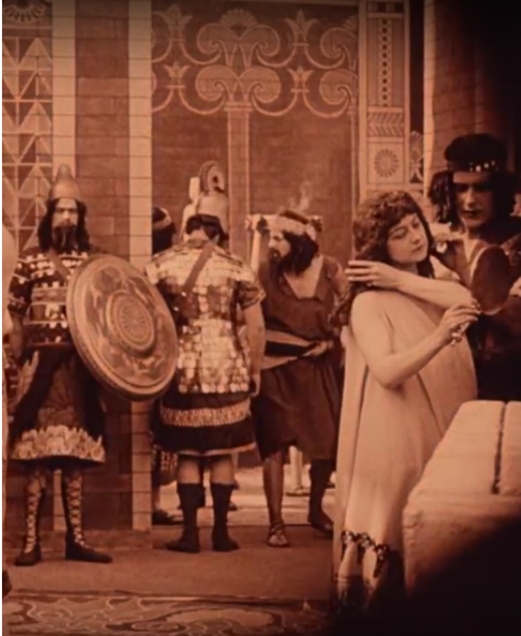
Fig. 5. Still from the movie Intolerance . Detail of the decoration of the back wall.
